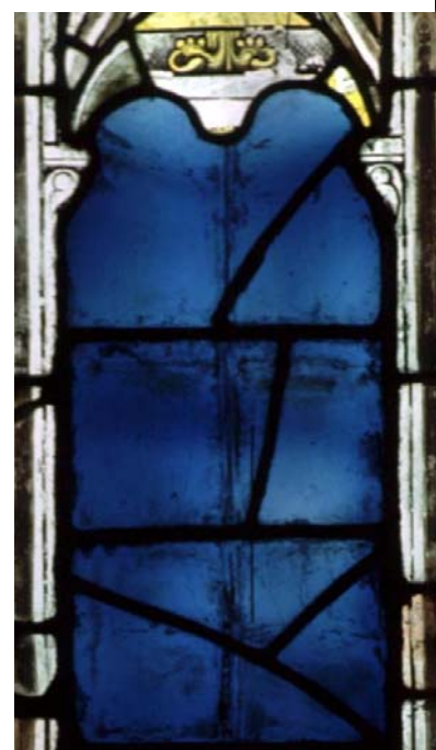
fig. 35 H3, 1 Corrosion line due to water run-off
