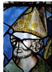
fig. 60 D4 Repair with unpainted glass
