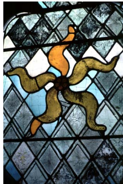
fig. 14 J3 Quarries replaced with unpainted glass
