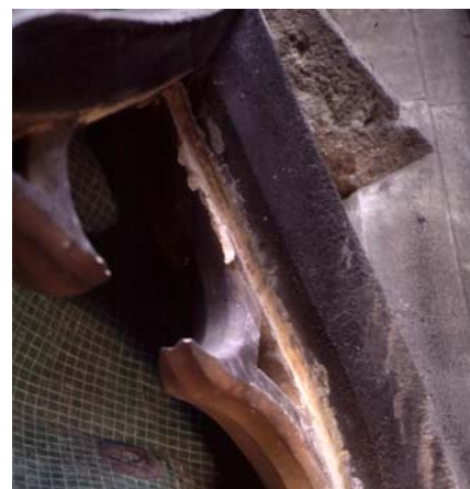
fig. 9 View of 'false' tracery in tier C, seen from the outside with the glass removed.
