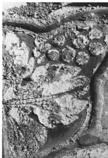
fig. 82 Weathering crust on the interior of a window from Erfurt. The well-preserved dark paint layer is beginning to fail along the edges.
