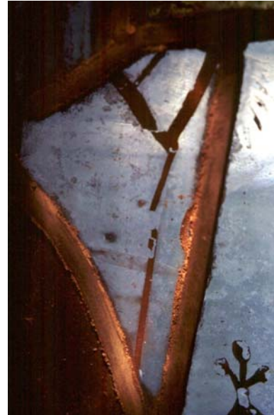
fig. 37 Dislocated paint flakes.
