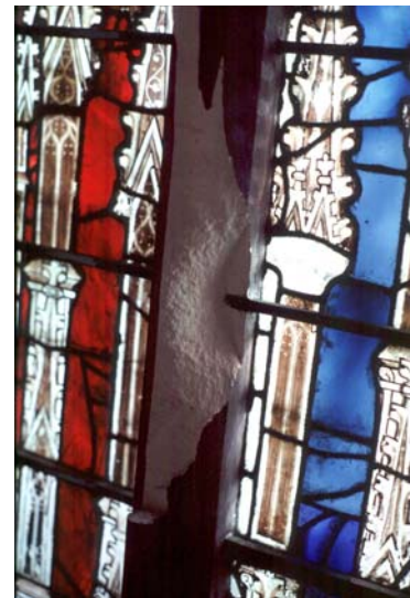
fig. 10 Damage to mullion by expanding ferrous saddle bar.
