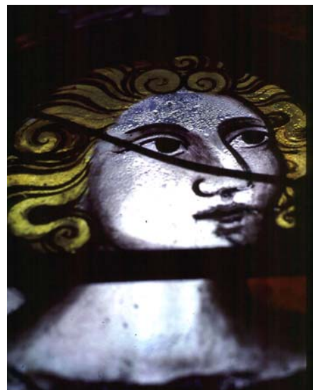
fig. 31 G4 Condensation on the internal surface of the Great East Window
