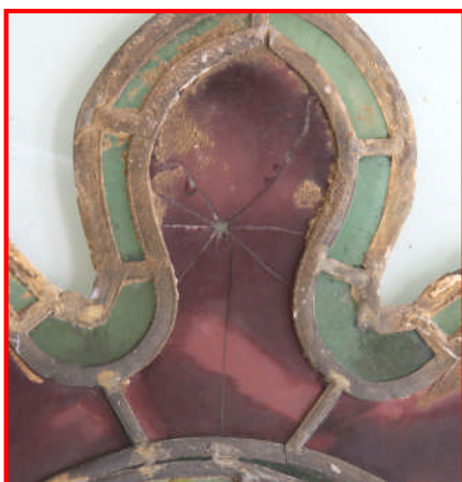
Impact fracture; putty remains; surviving back-painting
