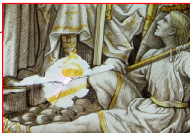
Impact fracture and shelled glass
