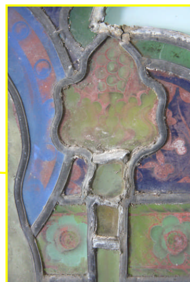
Previous repair: inserted stopgaps
