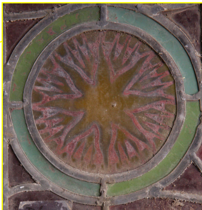
Surviving paint in poor condition
