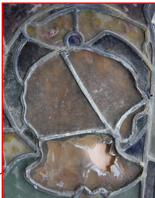
Damage and previous repair to head
