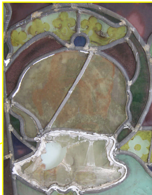
Previous repair insertion to head
