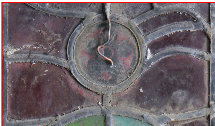
Copper tie; surface dirt
