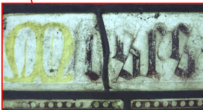
Variable loss of paint on inscription; break covered by strap lead
