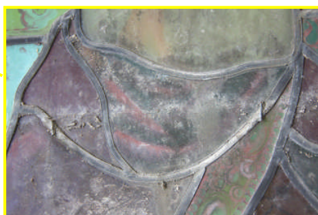
Surface dirt, remains of copper ties
