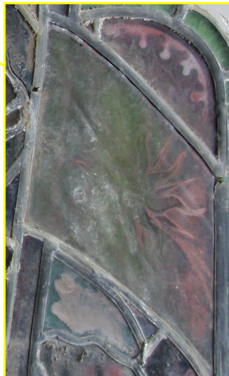
Surface dirt and some surviving paint
