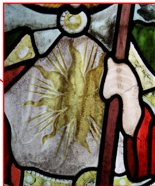
Surviving yellow stain but severe paint loss
