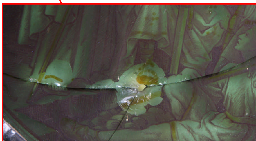
Impact fracture and shelled glass
