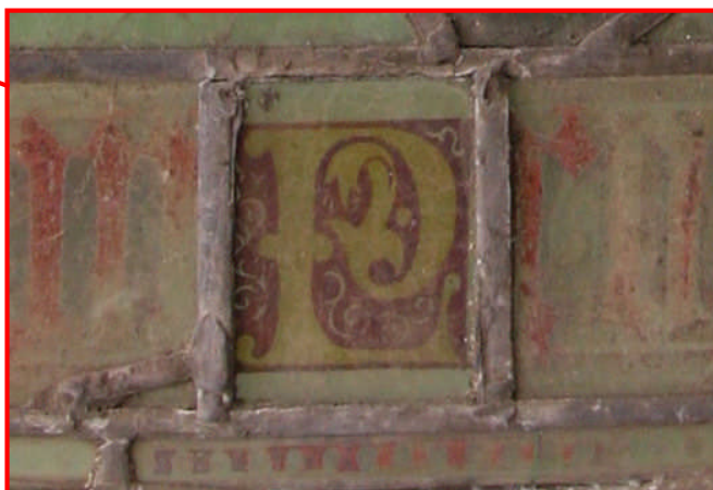
Inserted repair piece
