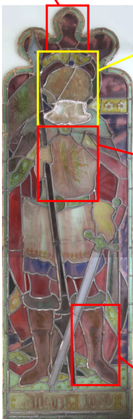
Impact fracture; putty remains; surviving back-painting
