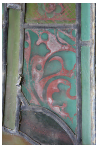
Figure 47: Detail of deteriorated paint on inside face (reflected light)
